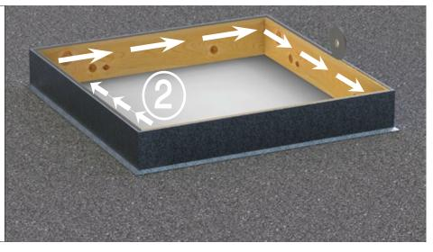
Mount skylight over curb and press down into seal. Secure skylight to curb with #10x2" wood screws through holes in flange of skylight.
