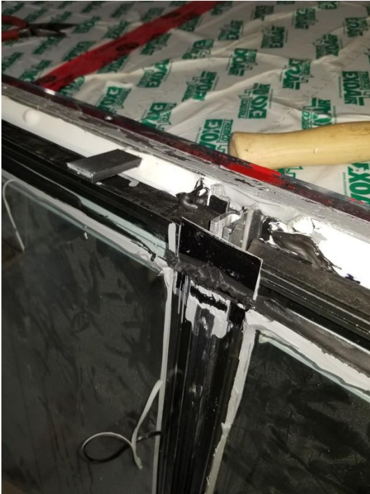
Photo 6- Aluminum plate at ends of pressure plate.
