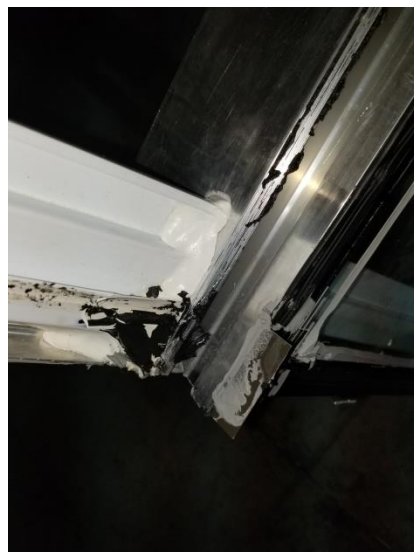
Photos 2, 3, and 4- Sealing of condensation gutters to rafter and curb frame.
