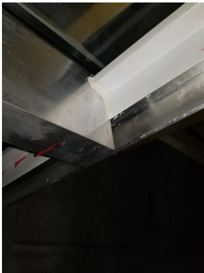
Photos 2, 3, and 4- Sealing of condensation gutters to rafter and curb frame.
