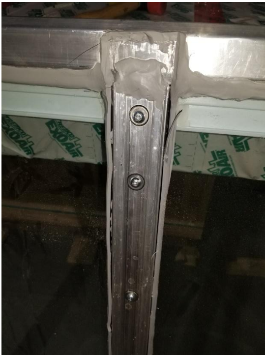
Photo 8- Cap bead of sealant at ends of pressure plate.
