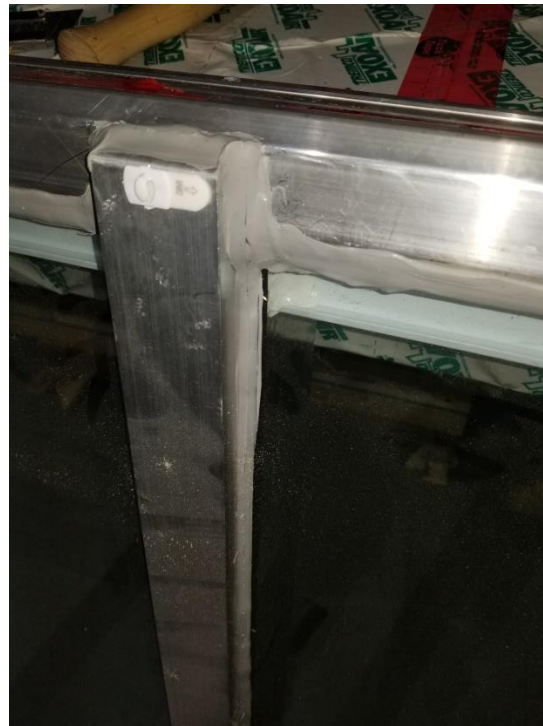
Photo 9- Cap bead of sealant on trim cap and retainer frame.
