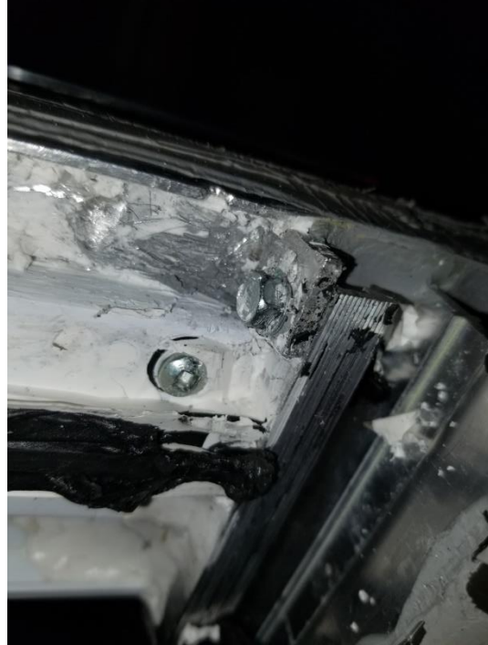
Photo 7- Angle bracket securing rafter.
